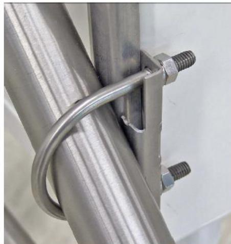
*Figure 7-9. The u-bolt bracket.*
